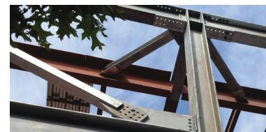
which use diagonal HSS8×8 braces that frame at three locations around the perimeter of the exoskeleton, two locations within the existing single-story section of the structure and three visually exposed locations at the new double-height interior atrium. The existing one-story building was laterally upgraded by tying it to the new two-story structure so that both behave as one.
