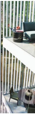
The house is conceived as two interlocking oppositional volumes: one highly transparent and oriented toward distant views and one solid and oriented towards the site. The taut transparent volume is delicately flanked at either end by a vertical steel screen of HSS6×2 columns spaced at 6 in. on center, which simultaneously and elegantly shades and structurally supports this portion of the house.
